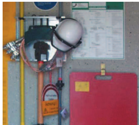
Pic. 16: Clamp for substation accessories and insulating protective barriers
