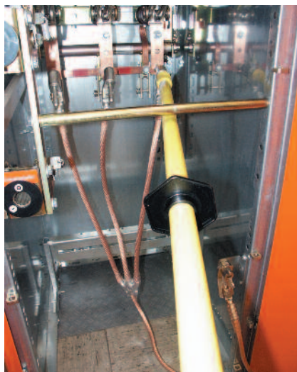
Pic. 12: Mounting of a earthing and short-circuiting device with a earthing stick
