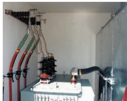
Medium voltage cable connectin cross-arm Steel parts hot galvanized
