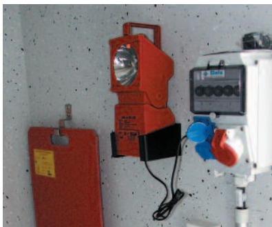
Pic. 18: LED-Hand emergency light in the wall-mounting holder and mounting for insulating protective barriers
