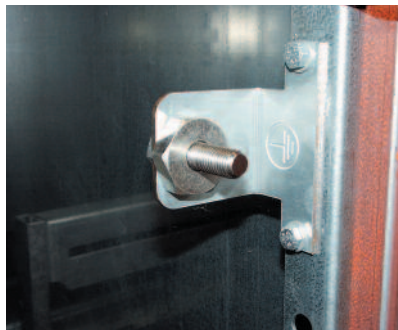
Pic. 9: Ground terminal studs
