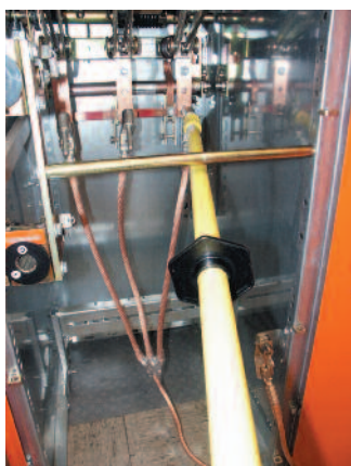
Pic. 2: Earthing stick while mounting of a earthing device
