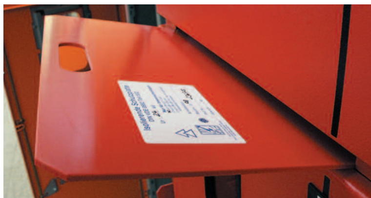
Pic. 14: Inserting of a protective barrier
